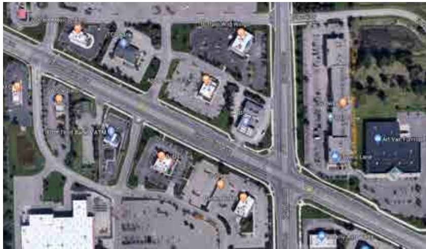
Shared driveway access and minimal curb cuts along Grand River in Genoa Township increases safety, traffic flow, and the overall appearance of the corridor.
